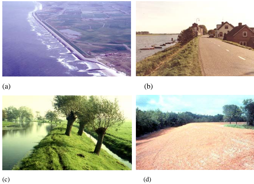
Figure 2.3: Dike along a (a) coastline, (b) river, (c) channel, and (d) on the floodplain.
