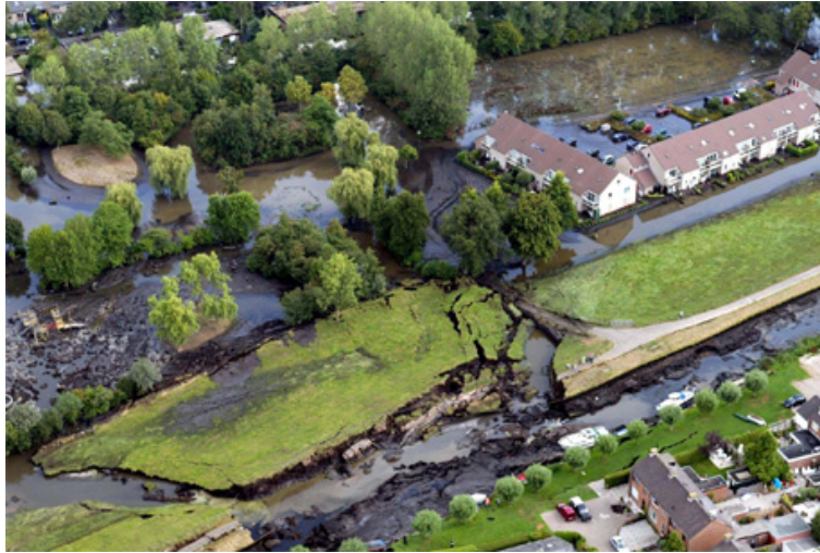
Figure 2.5: Failure of a canal dike in Wilnis, the Netherlands (2003).
