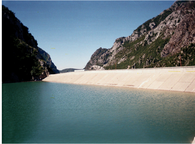
Figure 6.6: View of the Bovilla Dam facing upstream.
