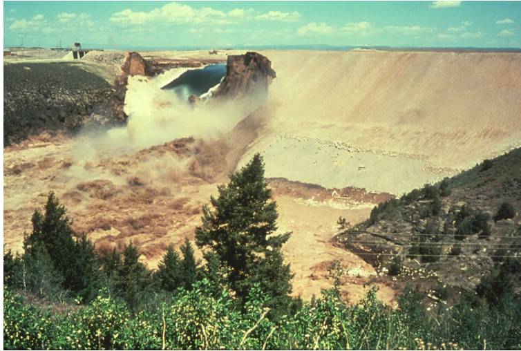
Figure 2.9: Teton Dam failure (Rogers, 2007).
