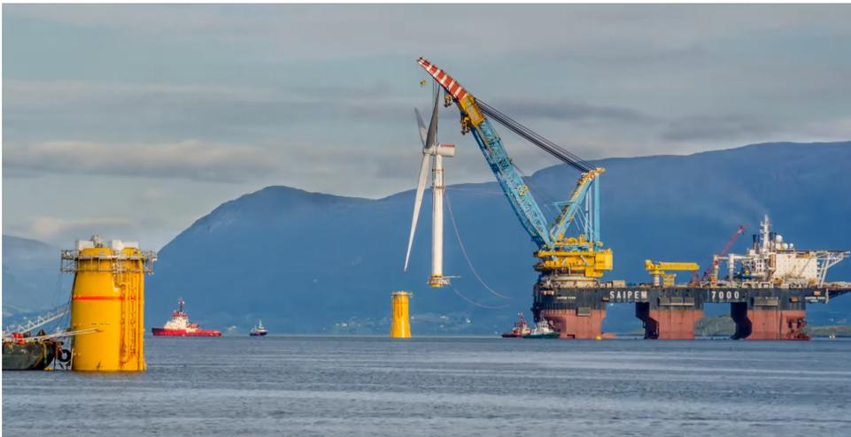
Figure 7.4: Mating of the tower-nacelle assembly with floating substructure (Håkonsen, 2017). Day rate for Saipem 7000 is around 630k€ (Bjørheim, 2015)
