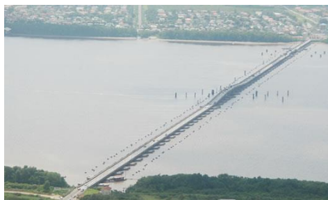
Demerara harbour bridge (Guyana) [6]
