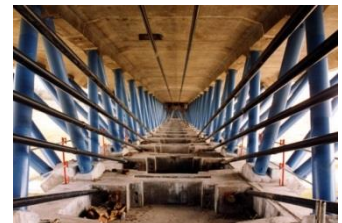
FIGURE 8-4 INSIDE THE ECHINGHEN VIADUCT [37]
