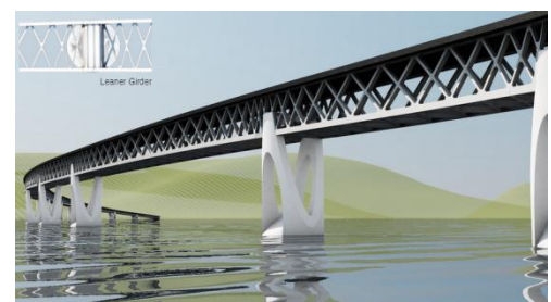
FIGURE 9-4 LATTICE BRIDGE GIRDERS [38]
