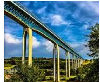
FIGURE 8-2 ECHINGHEN VIADUCT IN FRANCE [35]
