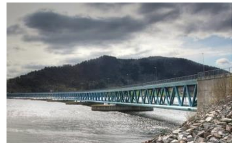
FIGURE A-3 BERGØYSUND FLOATING BRIDGE [5]
