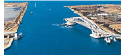
FIGURE A-7 YUMEMAI BRIDGE SWUNG OPEN [9]
