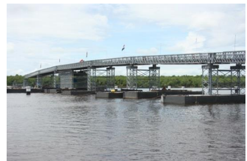
FIGURE A-2 BERBICE BRIDGE [4]
