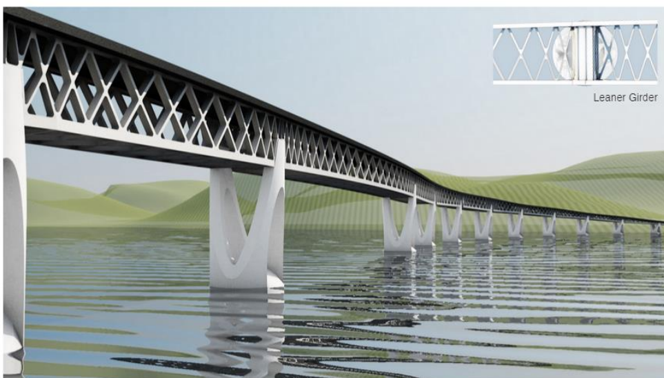
SOGNEFJORD BUOYANCY BRIDGE
