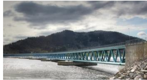
Bergøysund floating bridge (Norway) [5]
