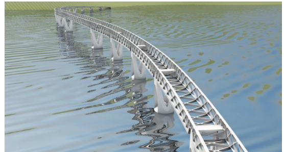
FIGURE 9-5 LATTICE BRIDGE GIRDERS WITHOUT THE TOP [38]
