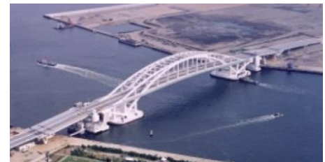
FIGURE A-6 YUMEMAI BRIDGE [8]
