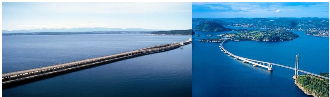
FIGURE A-1 CONTINUOUS PONTOON FLOATING BRIDGE (LEFT) AND SEPARATE PONTOON FLOATING BRIDGE (RIGHT) [25]
