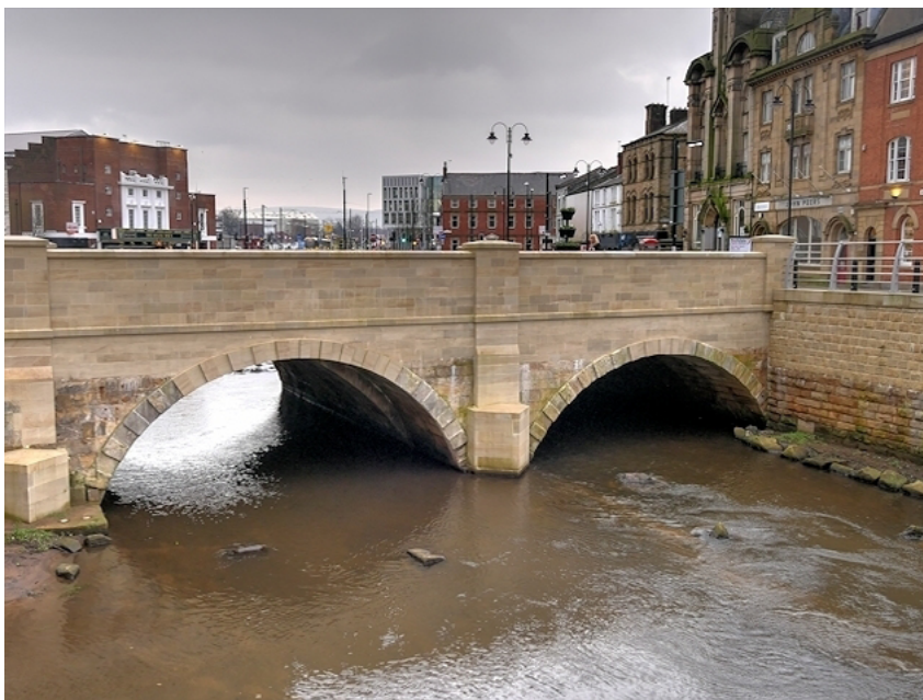
FIG. 6 Rochdale Bridge following restoration, 2017. Source: Copyright David Dixon and licensed for reuse under CC BY-SA 2.0 via geography.org.uk.
