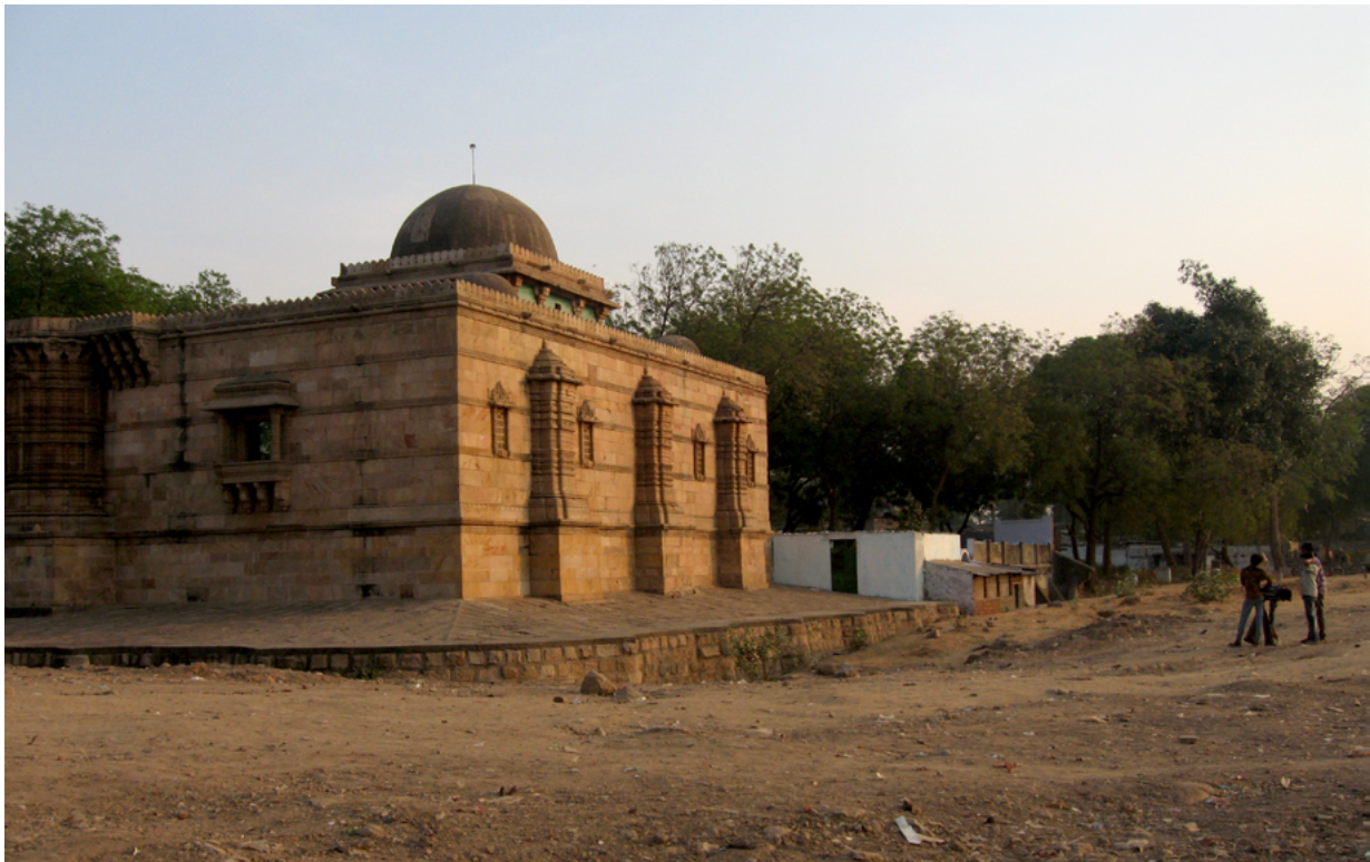
FIG. 16 Land reclamation and monument valorization on the eastern side of the Sabarmati showing also few remained shack houses (photo: Gloria Pessina, 2012)
