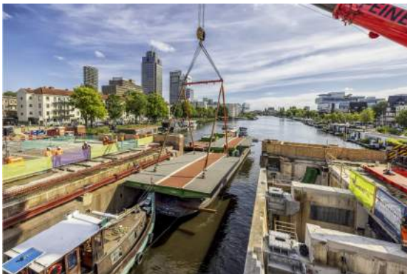
Figure G.1: A bridge leaf part being hoisted into place.
