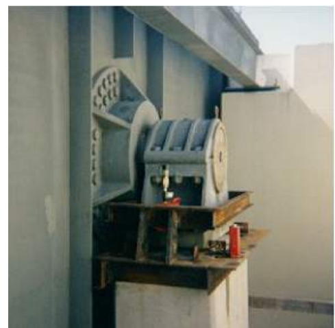
Figure 2.10: Trunnion support. (University of South Florida,2001)
