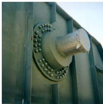
Figure 2.9: Reinforced connection element. (University of South Florida,2003)
