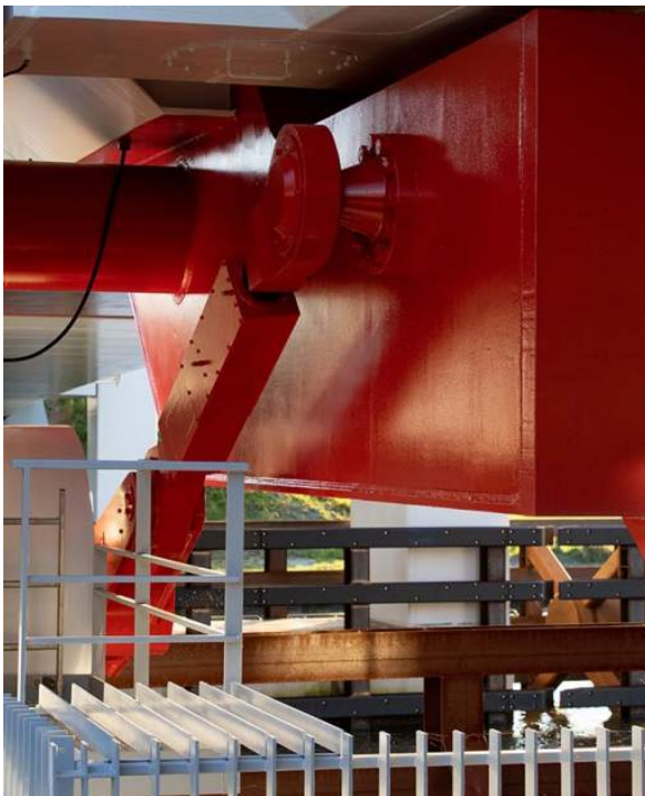
Figure 2.14: Hinged connection between push-pull rod and main beam. (ipv Delft, 2023)
