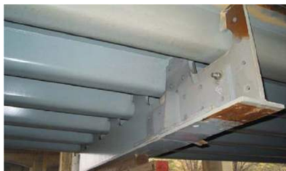
Figure 2.21: Connection between troughs and cross beams.(Connor et al.,2012)
