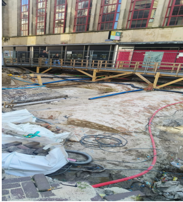
Figure 17: underground cables and wharf cellars
