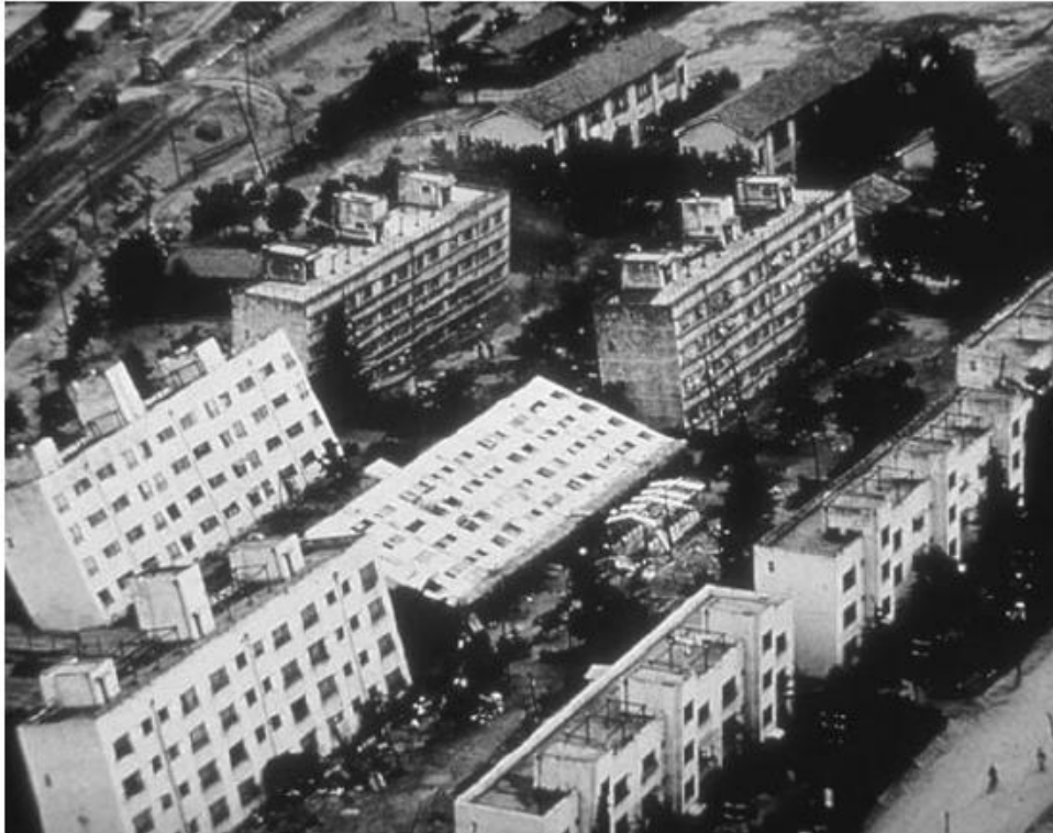
Figure 2.2: Foundation failure due to liquefaction, Niigata 1964 (Knappett & Craig, 2012)
