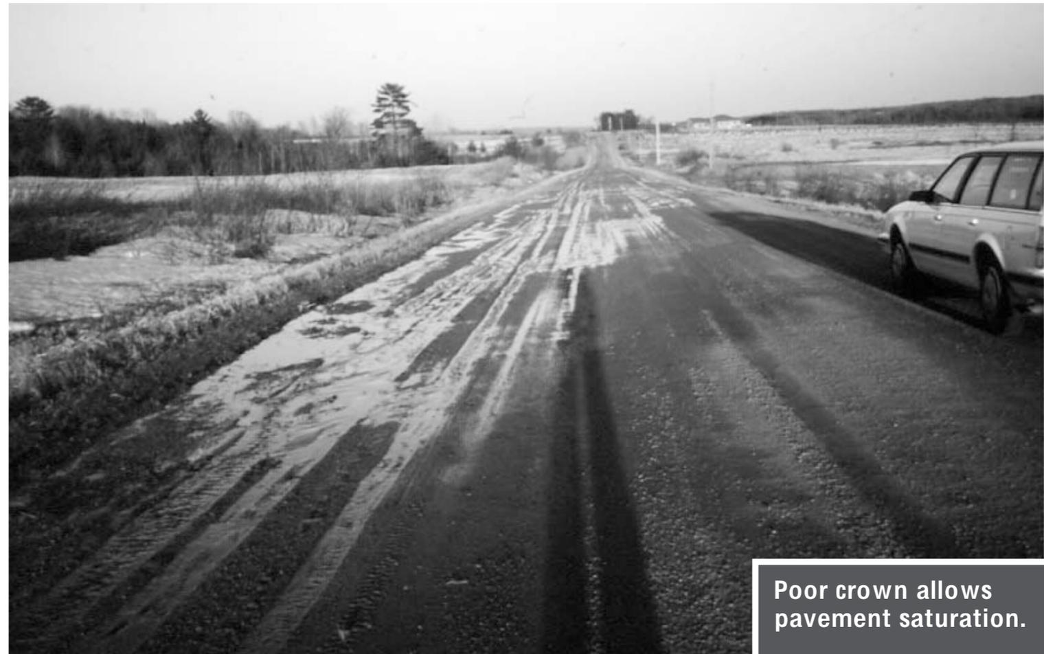
Poor crown allows pavement saturation.
