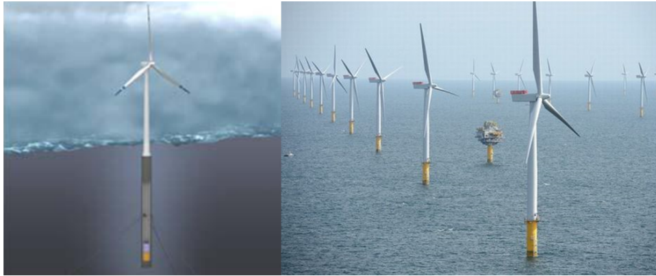
Figure 2.2: Example of an offshore wind park and a windmill floating support structure (Unknown, 2014)
