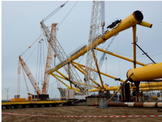
Figure 2.2: Assembly of Valemon jacket at Heerema Vlissingen yard. Source: www.hfg.heerema.com
