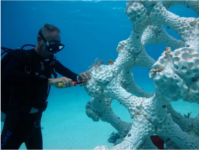
Applying coral samples to artificial reef by Coastruction | Fig. 18 (Piciocchi, 2019)
