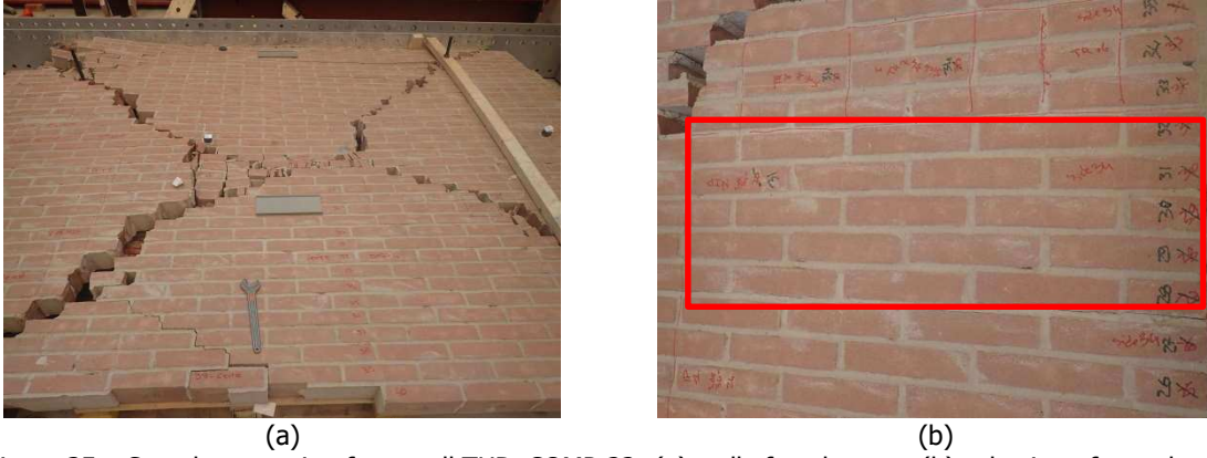
Figure 35 – Sample extraction from wall TUD_COMP-22: (a) wall after the test; (b) selection of samples to be sawn-cut for the in-plane bending.
