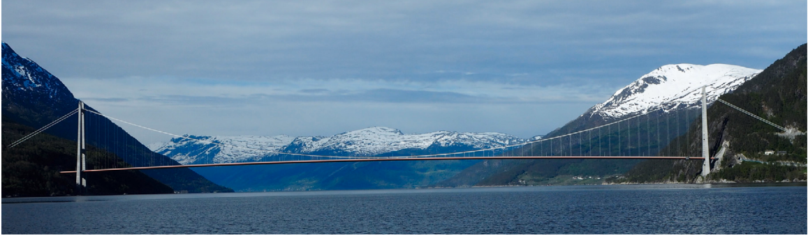
Fig. 3. The Hardanger Bridge (Photo: Aksel Fenerci/NTNU).
