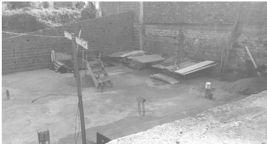
FIG. 6.29 Houses of bricks in the Favela do Telégrafo . Source: Ana Rosa Chagas Cavalcanti, 2015
