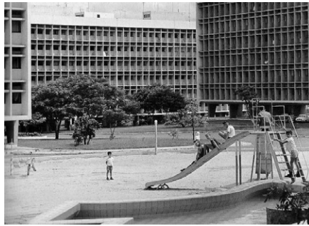
FIG. 6.7 Zoom of a Superquadra in the 1960s, composed by residential buildings with pilotis (stilts) and cobogós . Source: unknown.
