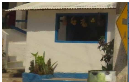
FIG. 6.18 "Window shop" in an informal house of a favela in Brazil. Source: Ana Rosa Chagas Cavalcanti, 2008;
