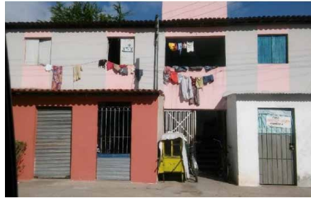
FIG. 5.10 Pictures show the housing project Vila S. Pedro six years later, 2016. Source: Ana Rosa Chagas Cavalcanti, 2016.
