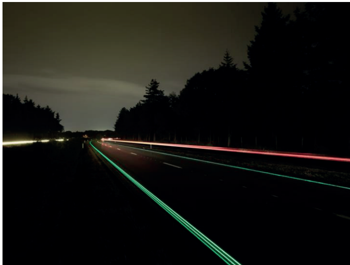
Figure 1.1. The glow-in-the-dark highway (N329) in the Netherlands. The figure is from Ref.12
