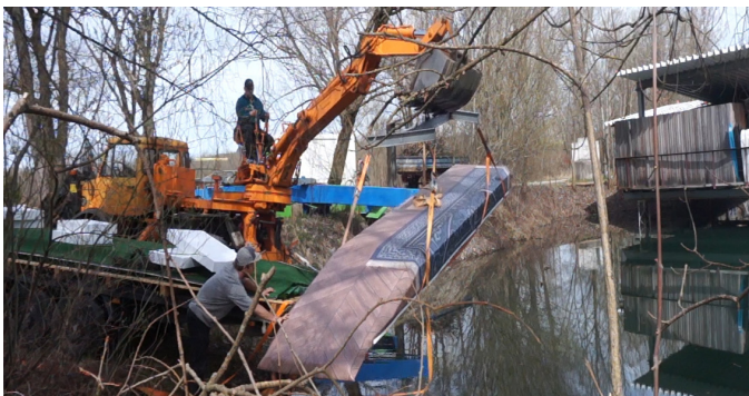
Figure 66: The prototypes were lifted into the lake using a crane.
