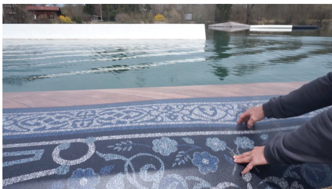
Figure 69: The PVC floor blew up like a balloon because of the radiation of the sun.
