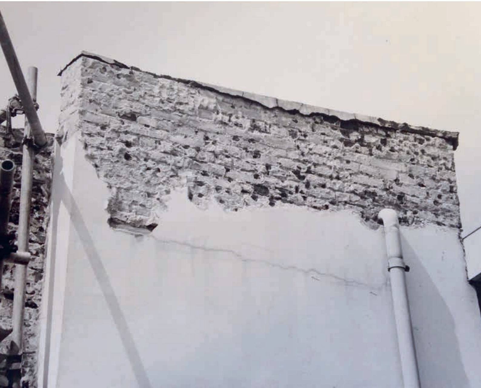
7. Only the render on the upper part of the white wall beside the front door of the Rietveld Schröder House was chipped away in 1979 (Bertus Mulder archive)
