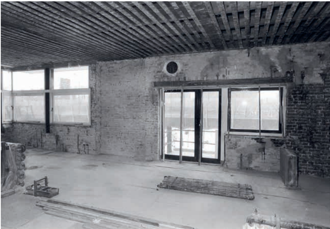
14. During the restoration of the upper floor of the Rietveld Schröder House in 1985-1986, Bertus Mulder completely stripped the walls and ceiling (Bertus Mulder archive)
