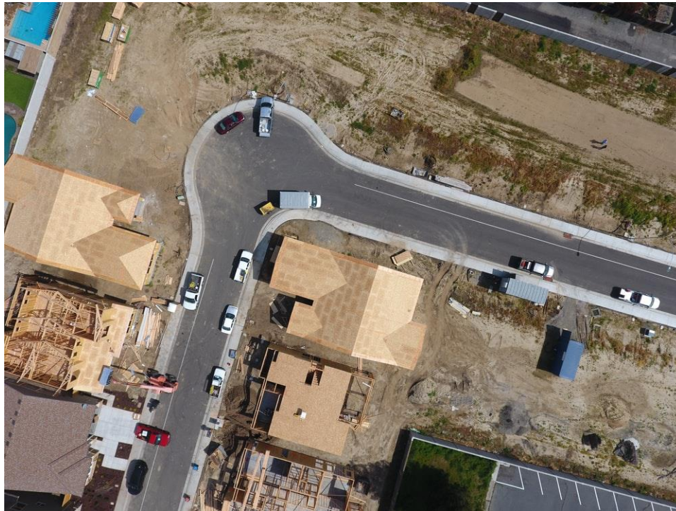
Neighbourhood construction. Source: Scott Blake on Unsplash.
