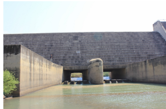
(b) Two uncontrolled bottom outlets
