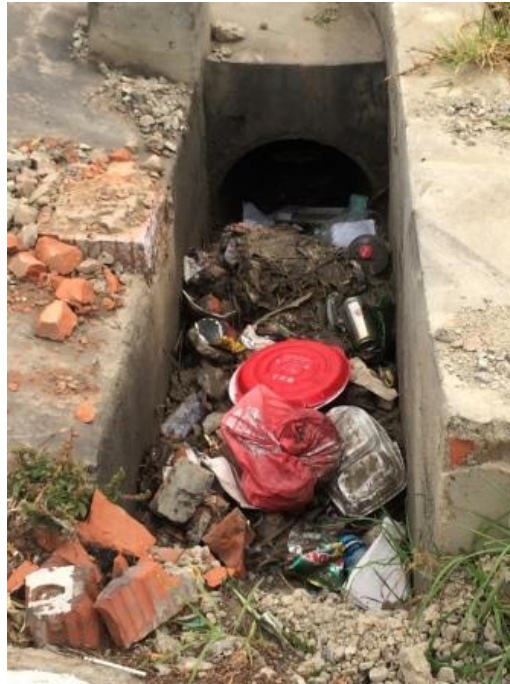
Figure 4.8: Blocked drainage inlet CBD Ladysmith
