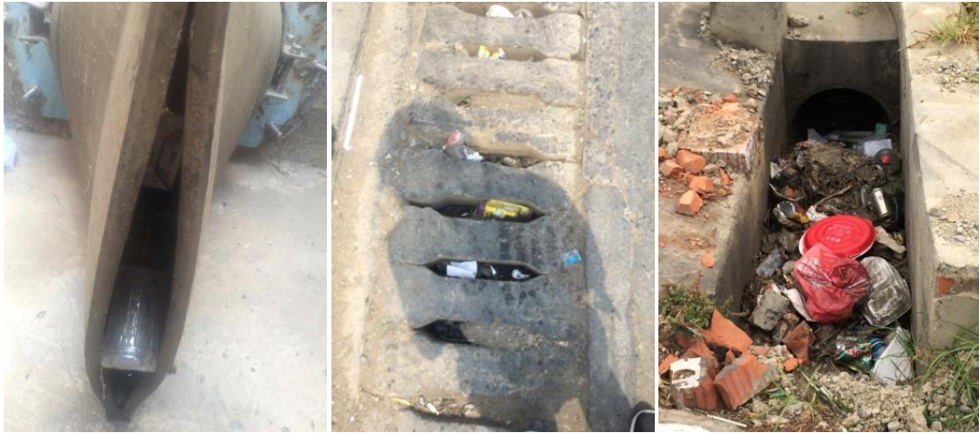
(a) Storm watervalue with debris
