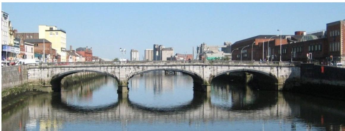
For bridges (and culverts), 'afflux' is an important hydraulic impact. Afflux is defined as the maximum rise in water surface elevation above that which would exist if the bridge was not there. It is most important in flood conditions.
