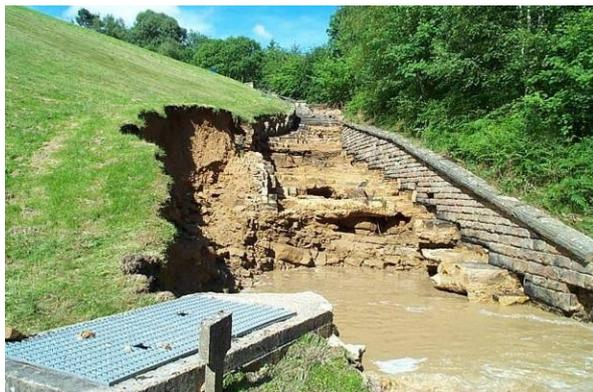
**Figure 7.7 High turbulence and frictional forces**
