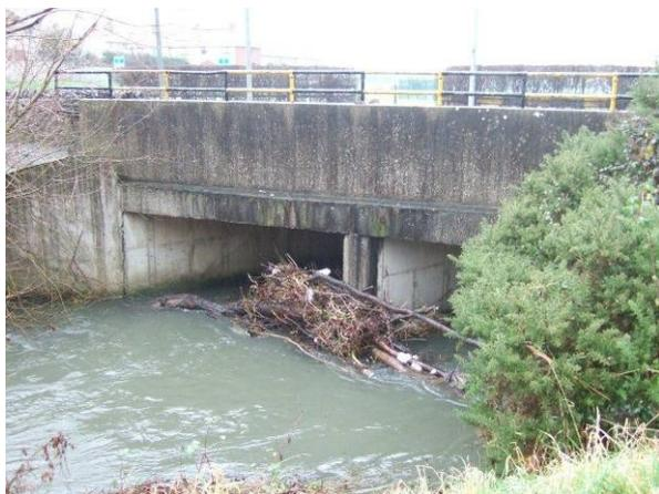
**Figure 7.19 Culvert blockage**
