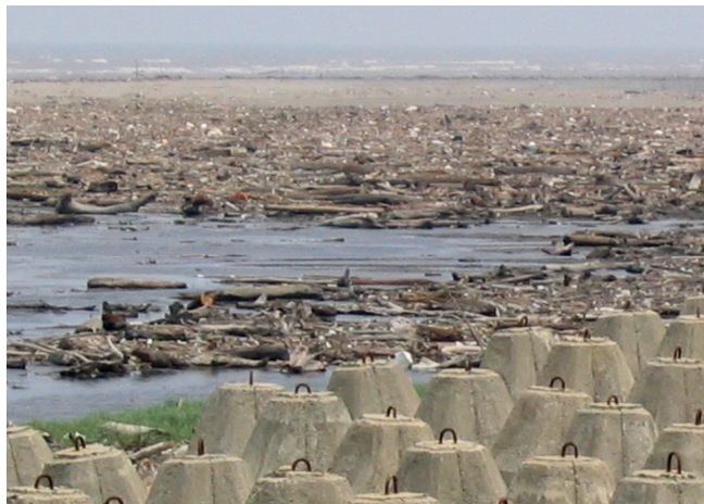
Figure 2.2 A plain outside the sea dike
