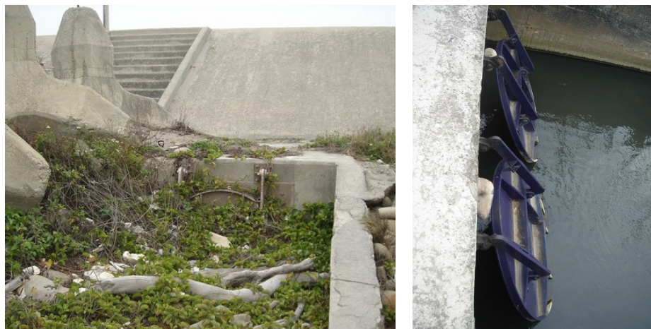
Figure 2.7 Two different outlet gate with stones or siltation
