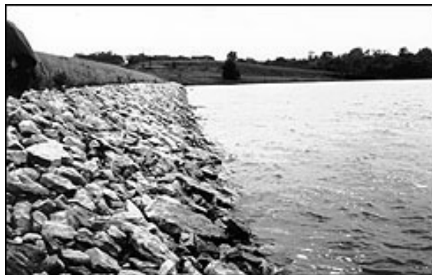
Figure 8.3 Example loose rock revetment
