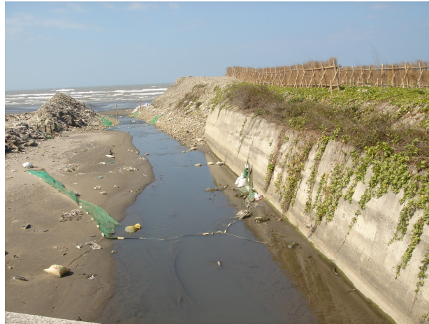
Figure 2.6 An outlet, with on the right screens of bamboo to prevent sand from being blown into it
