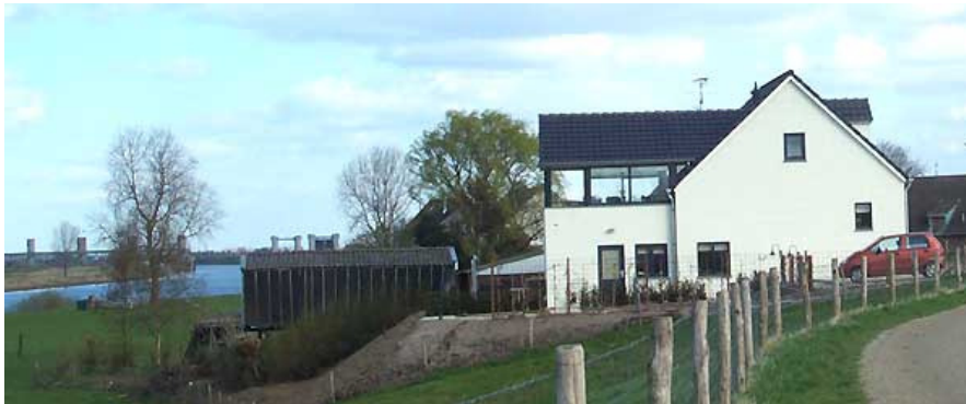
Figure 7.4 A residential building on a primary water defense
