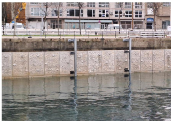
Figure 8.4: Seawall panels installed at the Port of Vigo (ECONcrete, 2024)
