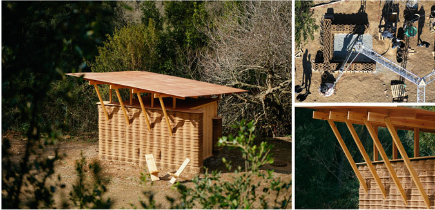
Fig. 7.4 TOVA (2022) is a completed circular building prototype using locally sourced materials constructed with 3DP processes achieved by a layer-based deposition of earth material mixture and a timber wood structure and a network of cavities in the wall that participates in the climate-responsiveness of the building. (Photographs by Gregori Civera)
