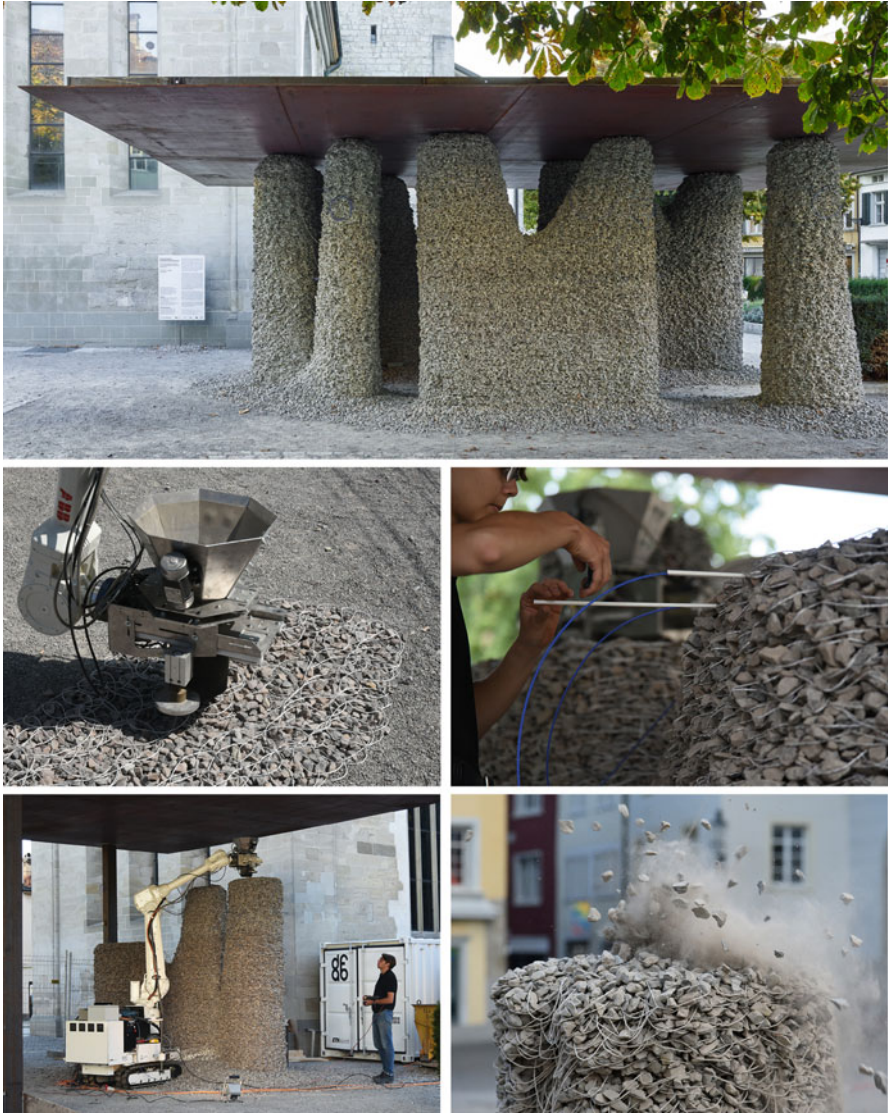
Fig. 9.1 (i) The Rock Print Pavilion is a full-scale robotically jammed structure composed of gravel aggregates and twine. The enabling technologies facilitating the on-site adaptive construction process include a custom robotic end-effector (ii) for extruding twine, depositing aggregates, and compacting layers, a structural health monitoring approach for the movement of the structure and the roof over time (iii), and mobility and localisation of the IF enabling the production of a larger structure on uneven ground (iv). The structure can be easily deconstructed with no material downgrading by removing the twine (v). (© Georg Aerni)
