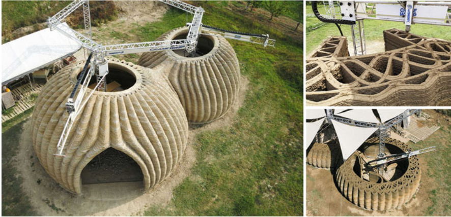
Fig. 7.3 The sustainable, innovative TECLA model (2021) of on-site housing construction uses materials sourced from the construction site and constructed using the modular Crane WASP machine. (© WASP)
