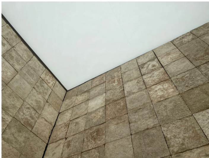
Fig. 15.1 The In Vivo Pavilion at the 18th International Architecture Exhibition in Venice. Mycelium, used as a regenerative building material, is kept alive so that the walls can self-repair
