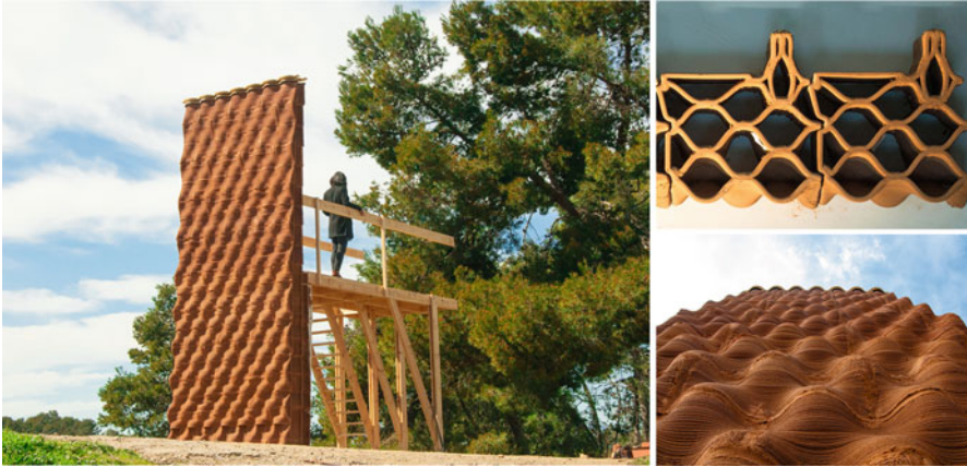
Fig. 7.2 Digital Adobe (2018) is the outcome of research on 3DPE for a performative habitat. Design parameters in robotic construction enhance climatic and structural properties innate to the material. Thermal properties such as transmittance are regulated by robot precision through the geometry design of the global shape, surface texture, and ventilating cavities. (© Dongliang Ye)
