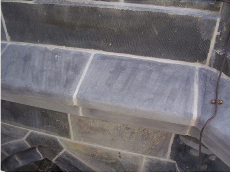
Fig. 5 Detail of the artificial patina on new sandstone at St. Lawrence Church Rotterdam (photo: T.G. Nijland)
