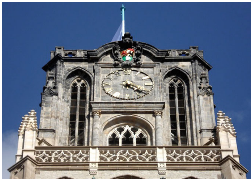
Fig. 4 Application of an artificial patina on new sandstone to visually match old sandstone at St. Lawrence Church Rotterdam (photo: W.J. Quist)
