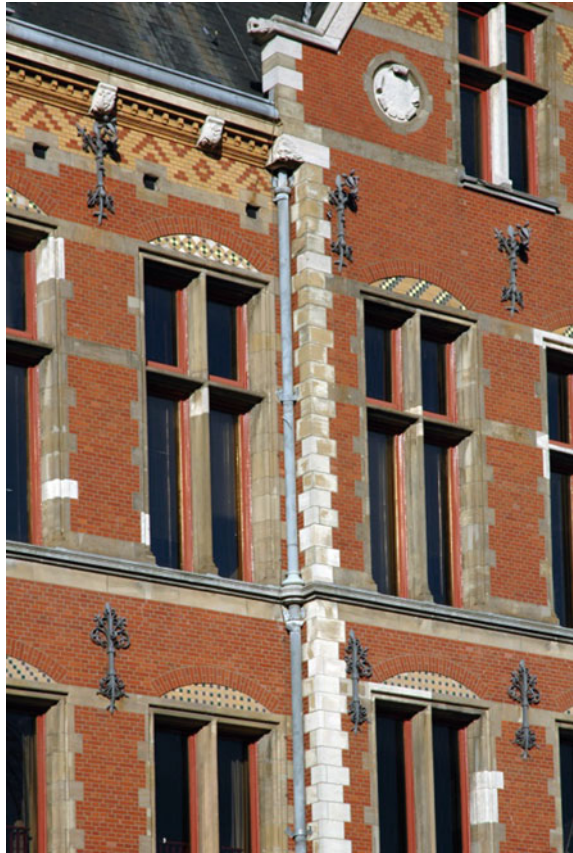
Fig. 7 The applied artificial patina on limestone at the Central Station of Amsterdam has been washed away by rain (photo: W.J. Quist)
