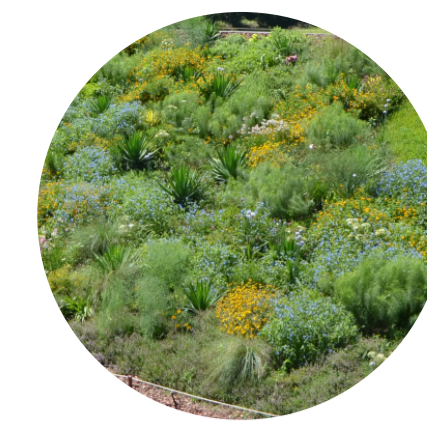
extensive roofs vegetation
