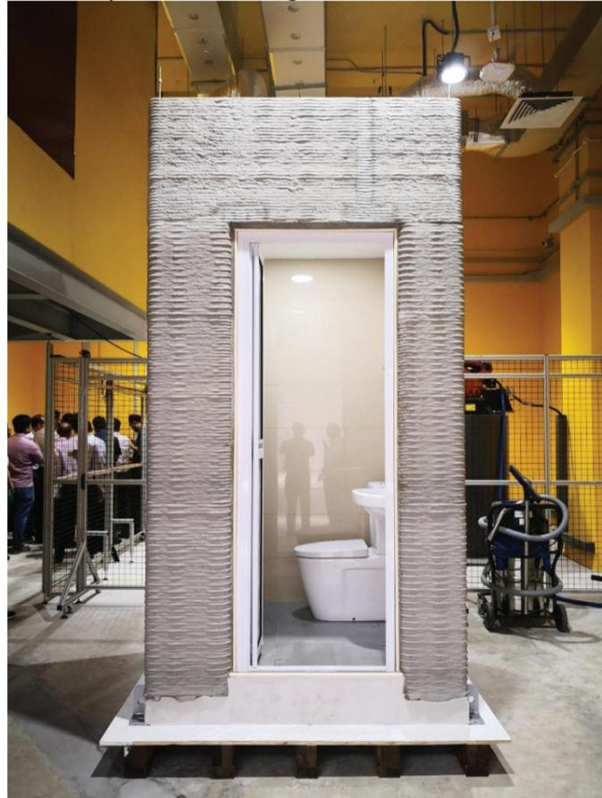
Image 4: 3d printed bathroom units (NTU)
