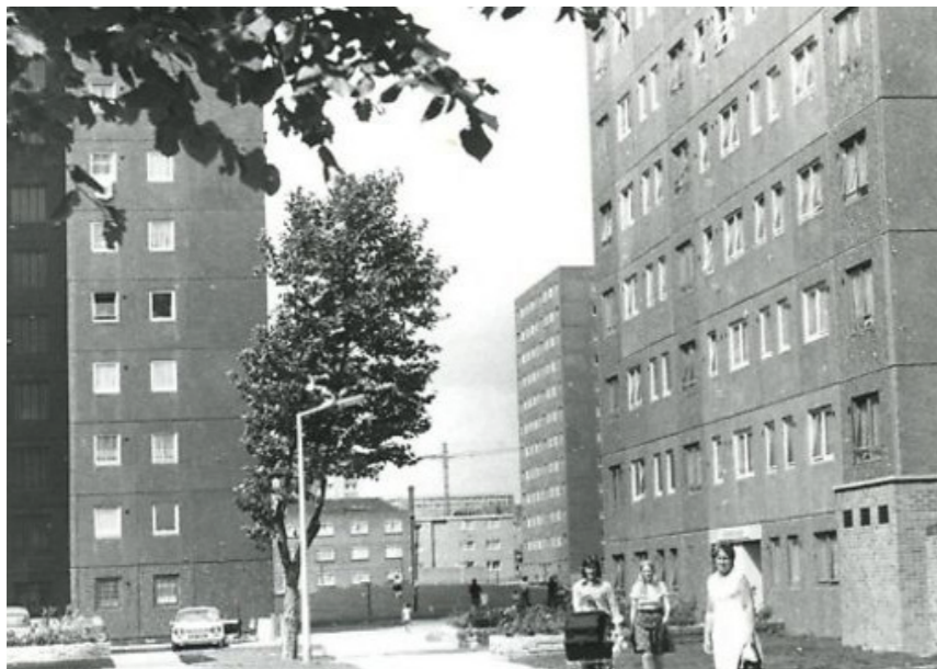
Figure 6.07 Highrise flats in the 1960s Richards, 2013
