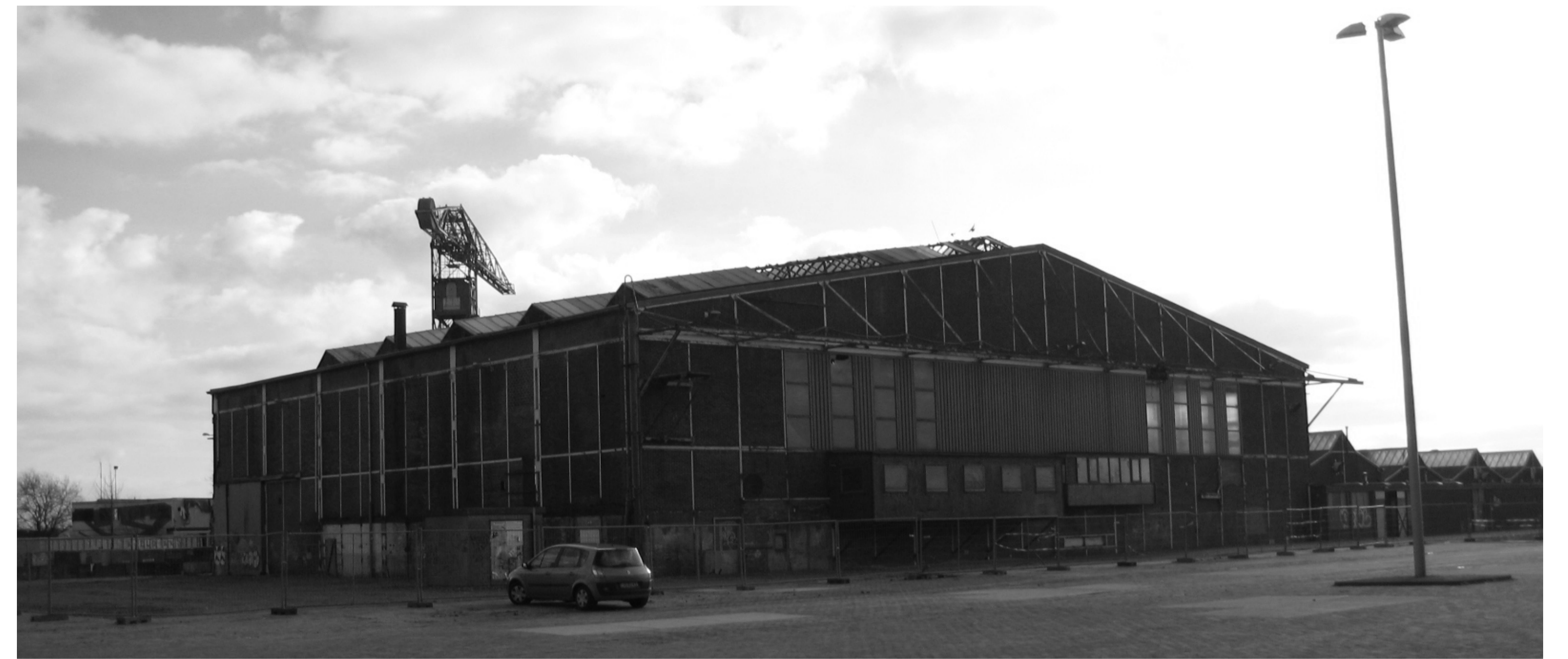
THE FORGING HALL
