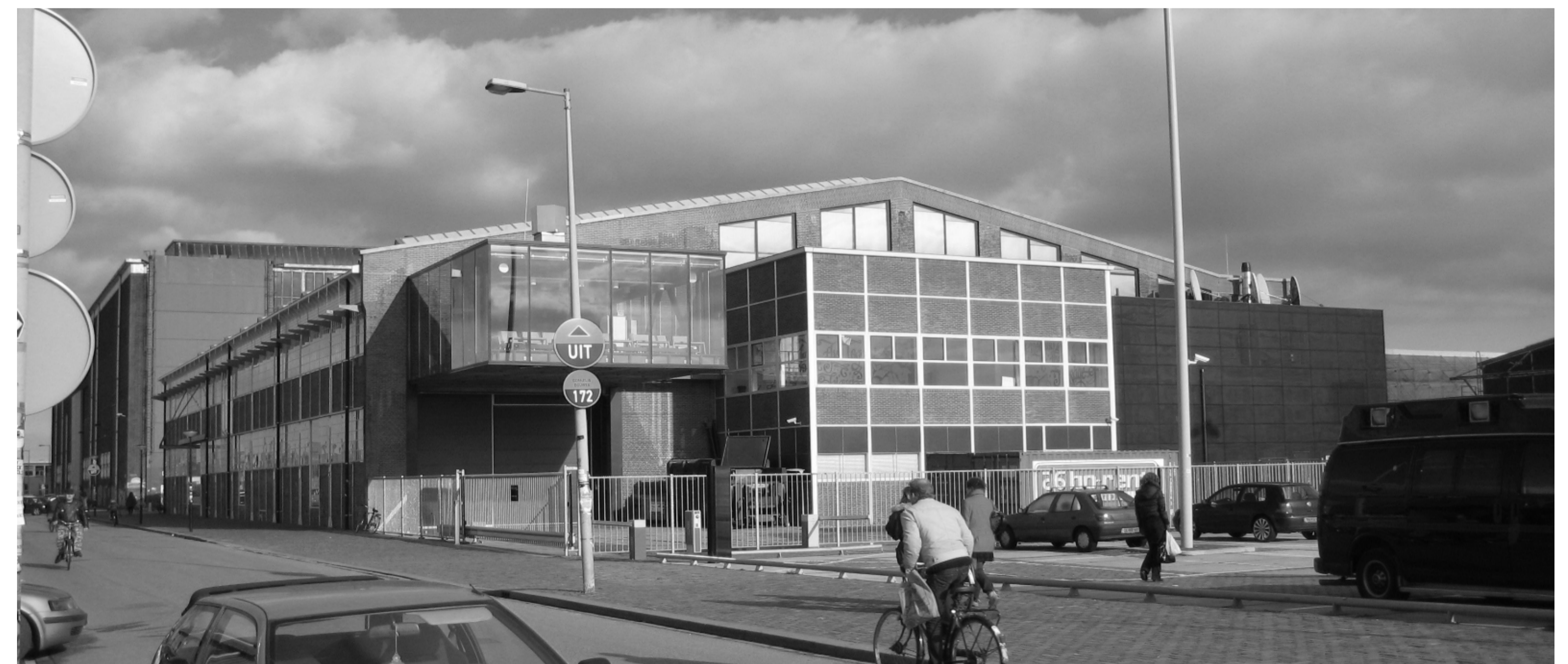
CARPENTING WORKSHOP- MTV BENELUX
