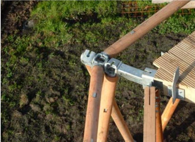
Figure 2.17: Connection implemented for the tower in Drenthe, The Netherlands by Tentech (P. A. d. Vries and Gard 2006).
