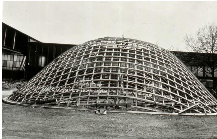
**Figure 2.28:** Trial gridshell, which is defined as a compression-only structure. It was built on a super-elliptical plan by Frei Otto in Essen, 1962 (Liddell 2015).
