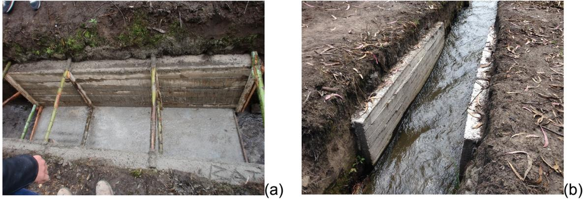
Figure 3: (a) Canal section 24 h after casting, (b) Five months after.
