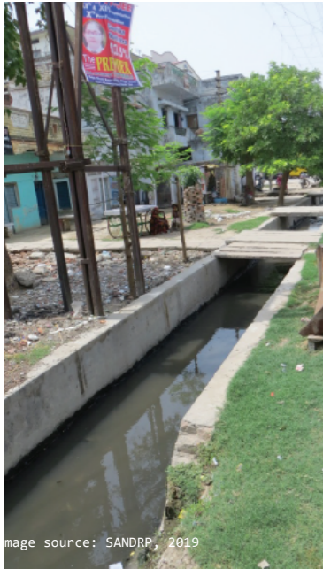
Open sewage drains
