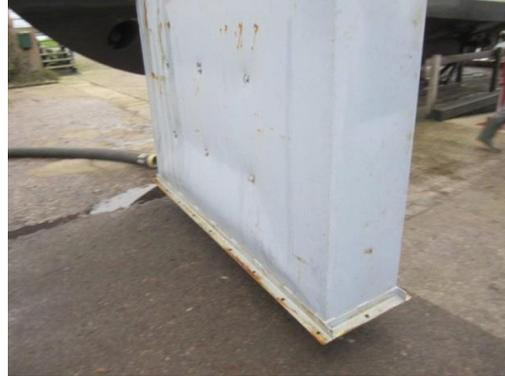
Picture 35. Bended lower module water column
