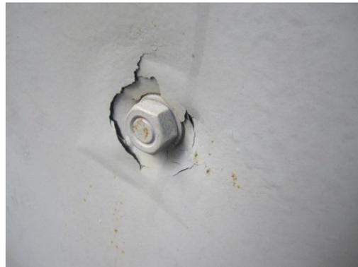
Picture 37. Broken epoxy paint by bending
