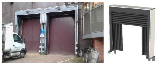
Figure 7.16a & 7.16b the current platform for loading and unloading the set and the potential saving dockshelter (Feldmann et al., 2016)
