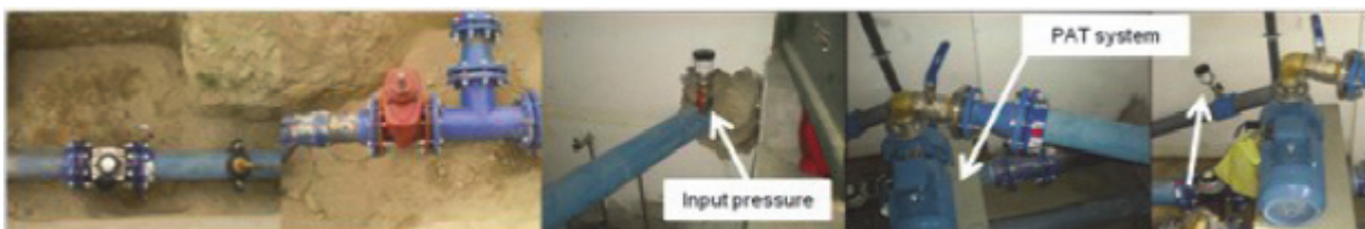
Figure 7-8: System tests in pipes
