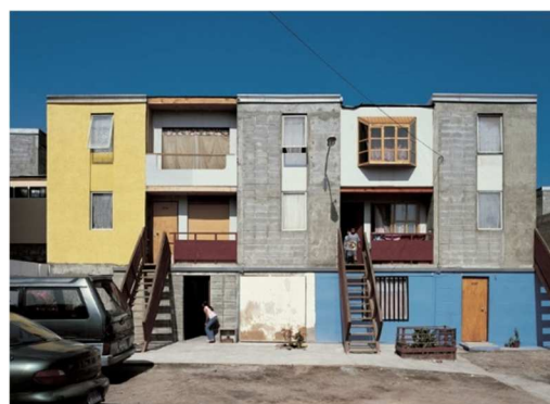
Figure 10 – Over time, and depending on their needs, the inhabitants changed their dwelling unit.
