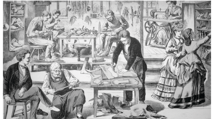
Fig. 2: The workshop and shop for customers on the ground floor
