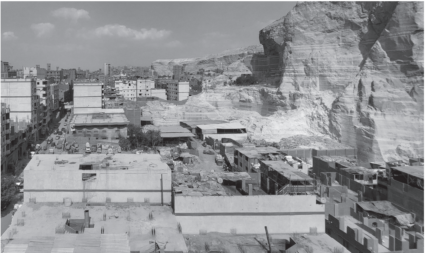
View from the pigeon tower to the north on the parking lot
