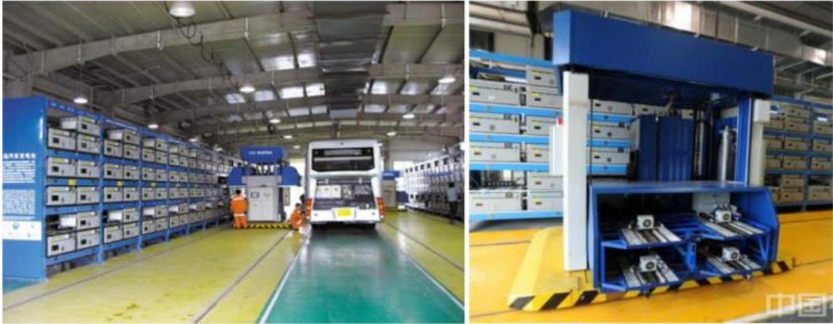
Figure 2-7 - Beijing's battery swapping station and quick battery exchange robot. Sources: Busworld (2013), Chao & Xiaohong (2013)
