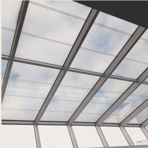
Onyx Solar HR+++ transparent BIPV panels
