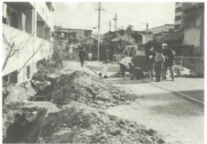
Photo 20 Apartment building sewer being repaired
