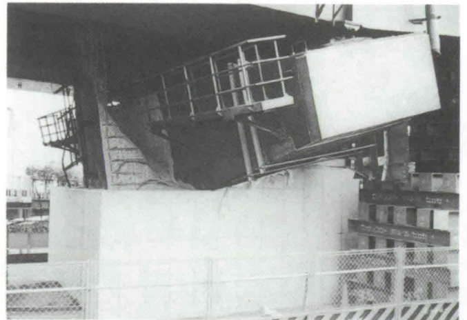
Photograph 6 Preventing the collapse of concrete viaduct pier (2)
