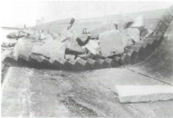
(c) Collapse of dike
