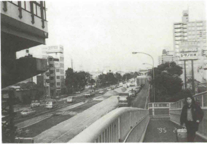
Photograph 1 National Highway Route 43 (Near Fukae)
