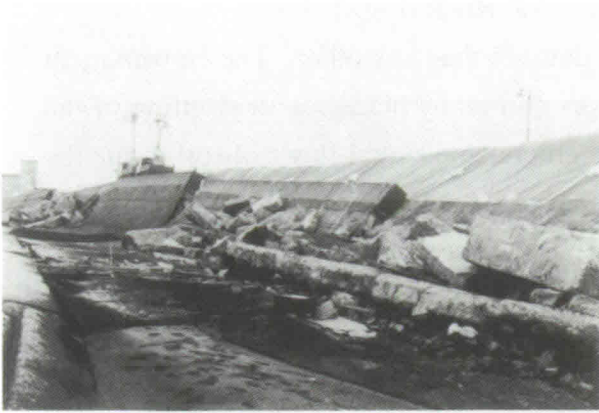
(a) Collapse of dike
