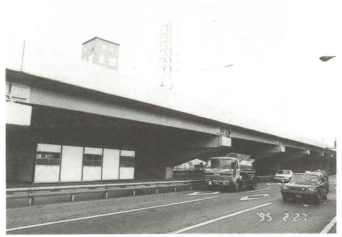
Photograph 16 Near Toyonaka-Minami Interchange ("No-Joint Method")
