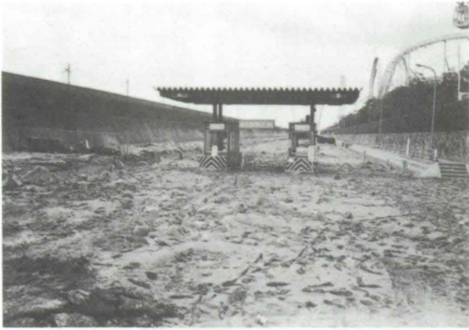
Photo 13 Liquefied soil on Port Island
