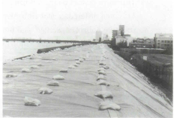
(b) Emergency repair work
