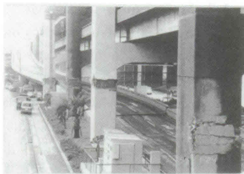
Photo 15 Collapsed RC bridge columns of moment frame structure at an approach to the Kobe-Hashi Bridge
