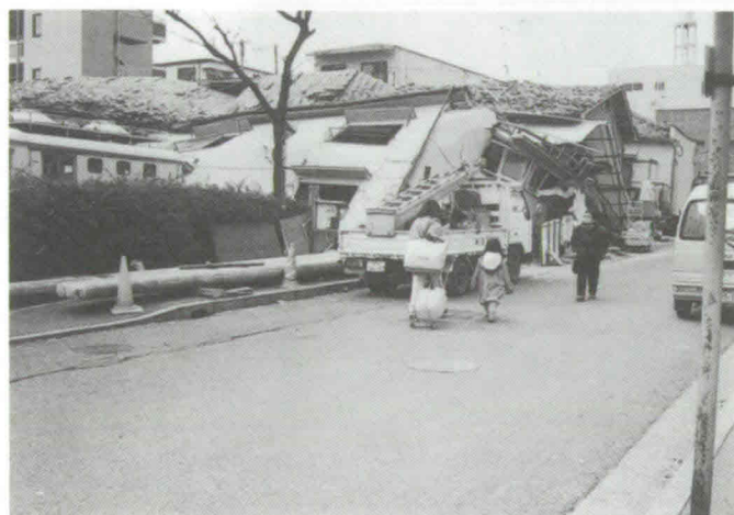
Photo 27 Water distribution point
