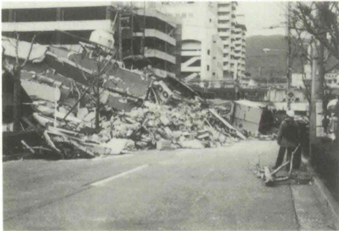
Photo 1 Street rendered impassable by the collapse of a parking building (at West Japan Railway Company's Ashiya Station)
