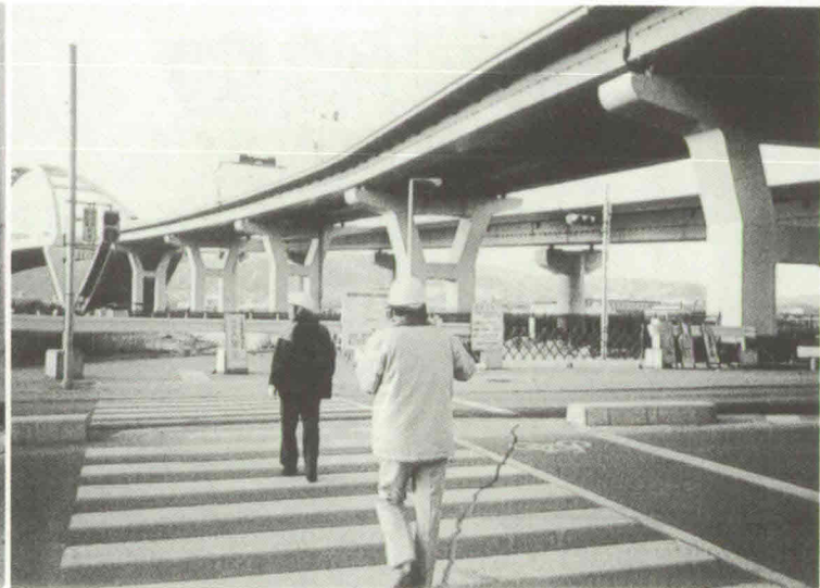
K11: Sound steel bridge pier supporting the Wangan Route
