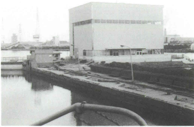
Photo 1 Liquefaction occurred around the Amagasaki Lock
