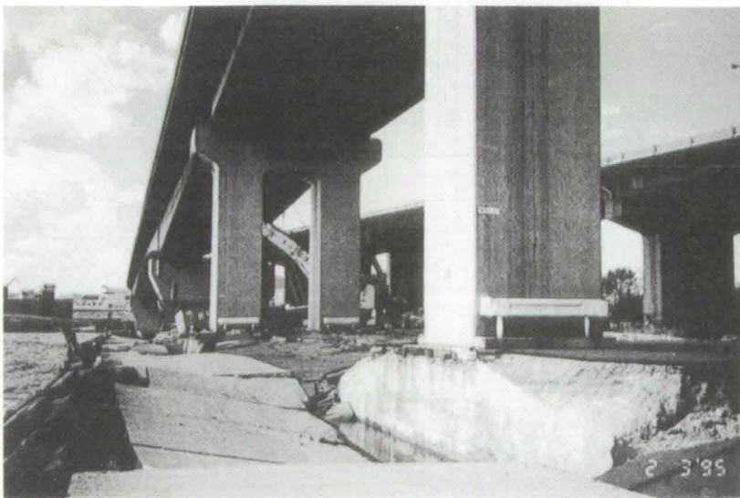
H16: Sound rigid-frame bridge piers
