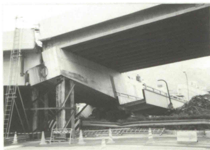
Photo 22 Collapsed steel T-shaped road bridge pier; RC T-shaped road bridge piers both before and behind also overturned (at the grade separated crossing of National Highways 43 and 2, Iwaya in Kobe)
