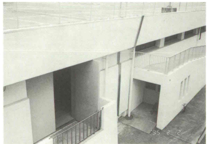
Photo 12 Port Island Sewage Treatment Plant
