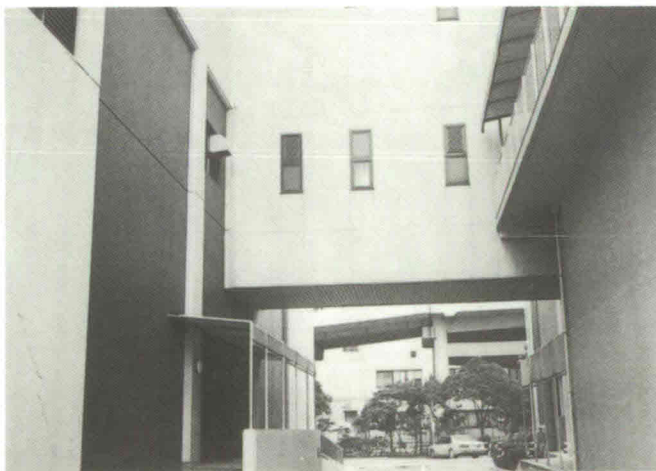
Photo 11 Port Island Sewage Treatment Plant
