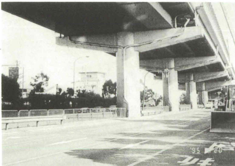
K1: Single-column circular bridge pier supporting the Hanshin Expressway
