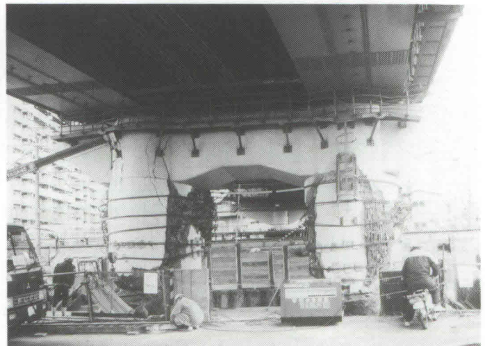
Photo 14 Failure of piers of the Second Shinmei Overbridge, with continuous steel box-girder superstructure
