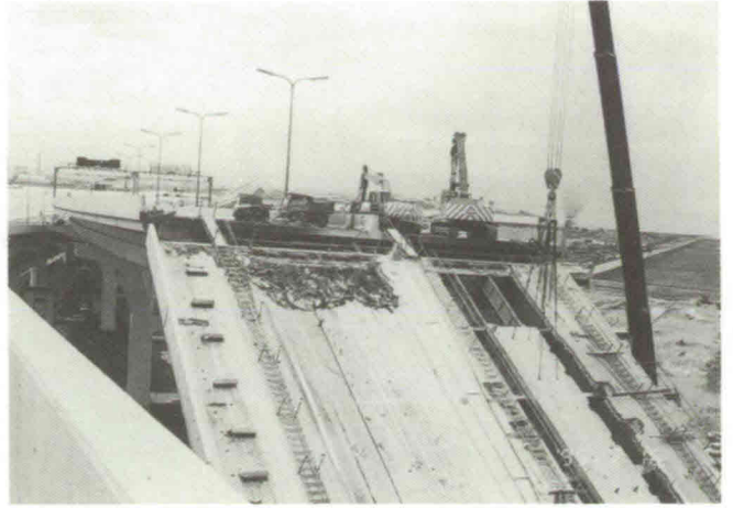
Photograph 12 Removal of floor slabs on side span of Nishinomiya Port Bridge
