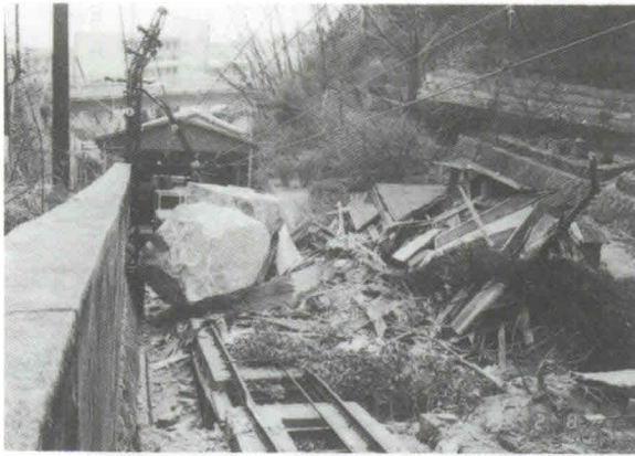
Photo 1 Rockfalls at Dobashi station, Rokko Cable Way
