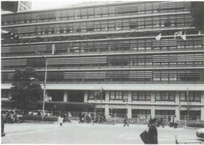
Photo 1 Damaged No.2 Building of Kobe City Office
