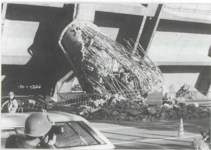
Photo 5 Overturned Pilz-type RC elevated expressway (Kobe Route in Fukae District)
