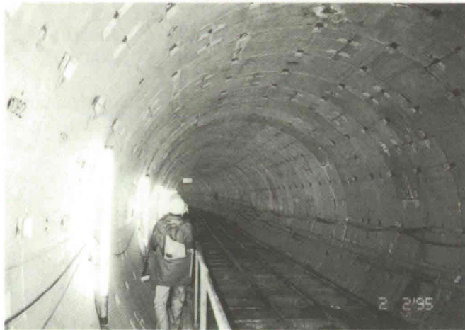
Photo 11 View of Kansai Electric Power Company's Isobe Dori Shield Tunnel
