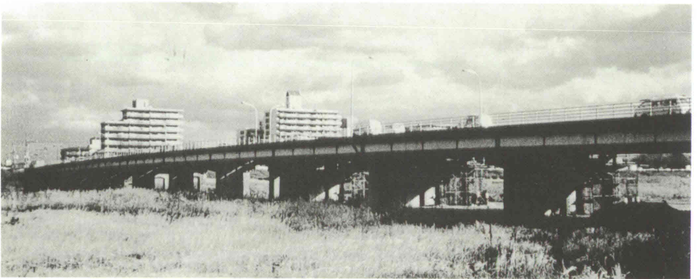
S12: Bridge piers supporting National Highway 171 with minor damage
