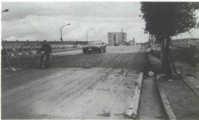
Photo 1 Laying asphalt mixture on road surface behind abutments
