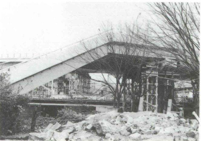
Photograph 9 Prevention of superstructure fall-off (2)
