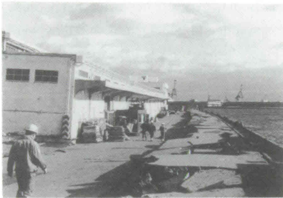
Photo 3 Damaged west quay of No. 6 Shinko jetty
