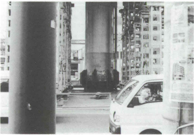
Photograph 7 Steel viaduct pier under repair
