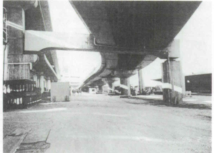
Photo 11 Piers of the elevated approach span connecting to the Kobe Bridge
