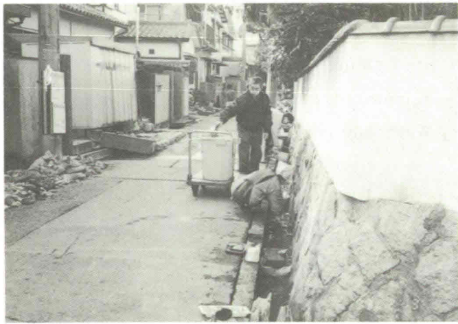
Photo 33 Citizens ladling leaking water from supply pipe
