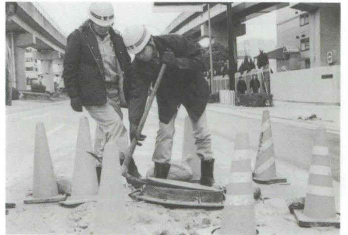
Photo 18 Survey of sewer pipes
