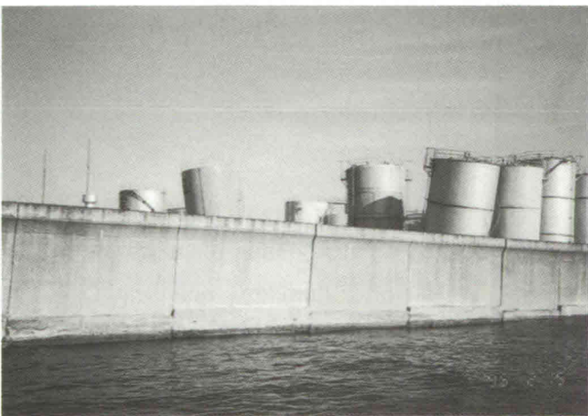
Photo 11 Tilting of small oil tanks in the Nagata Port
