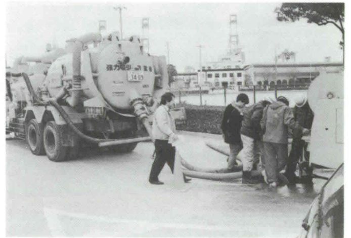
Photo 16 Survey of sewer pipes
