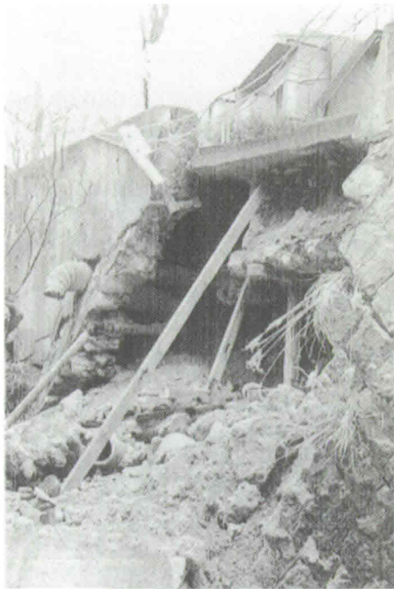
Photo 4 Collapsed fill at Okamoto 6-chome
