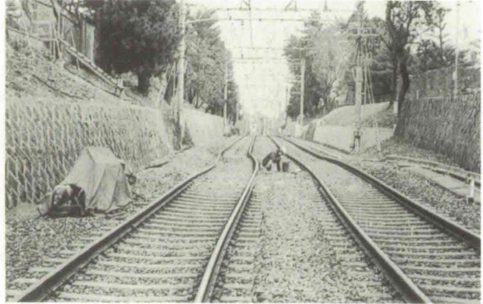
Photo 10 Landslide at Iwazono-cho
