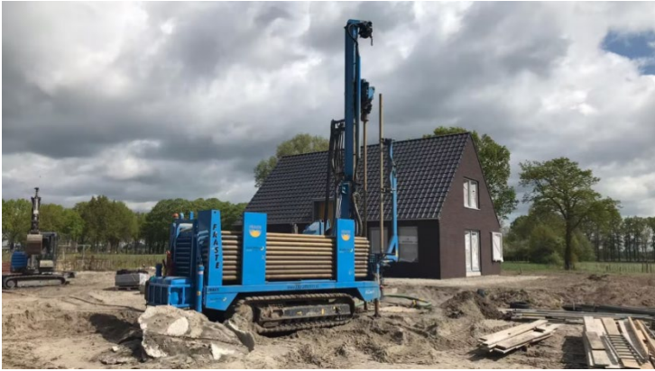
Figure 60. Back garden ground source drilling
