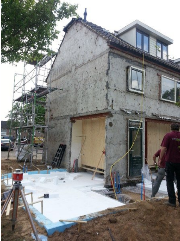
Figure 90. Private home Den Bosch NOM outer leaf demolished
