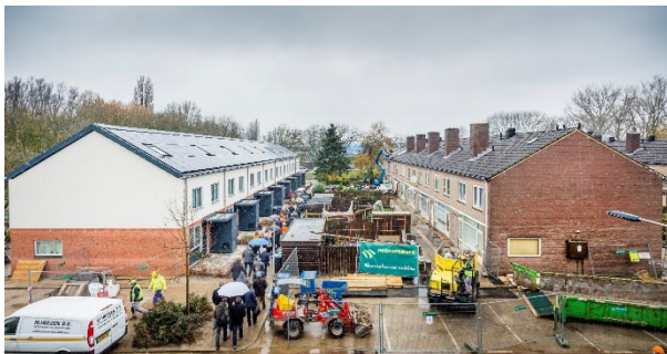
Figure 83. Presikhaaf NOM, left after and right before renovation
