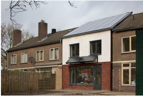
Figure 84. Presikhaaf NOM, before and after renovation
