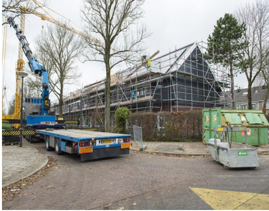
Figure 80. Woonwaard NOM renovation, envelope renovation
