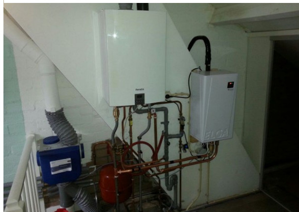
Figure 19. Hybrid air source heat pump + gas boiler + central heating buffer (Korbee, n.d.)
