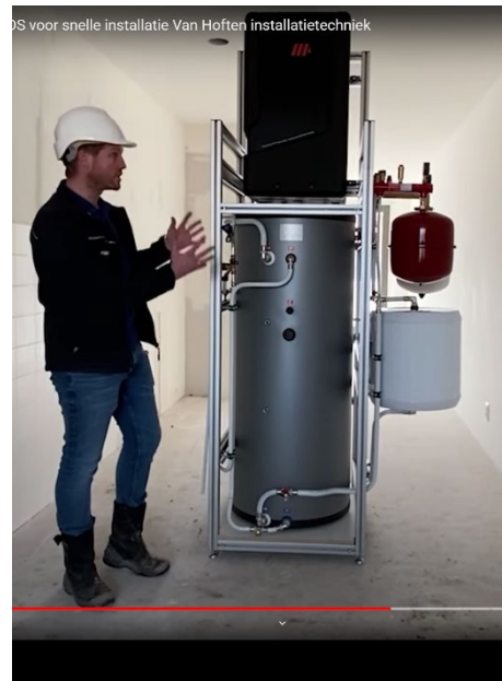
Figure 23. PVT heat pump indoor unit + DHW boiler + central heating buffer (Youtube)
