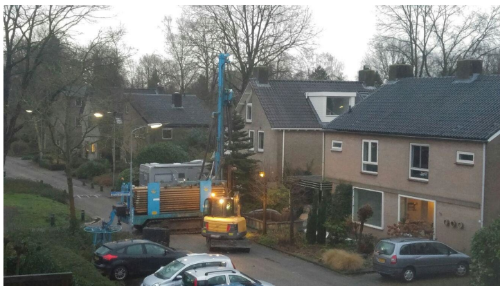
Figure 59. Front garden ground source drilling
