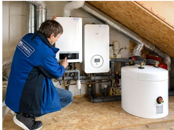
Figure 19. Hybrid air source heat pump + gas boiler + central heating buffer (Korbee, n.d.)
