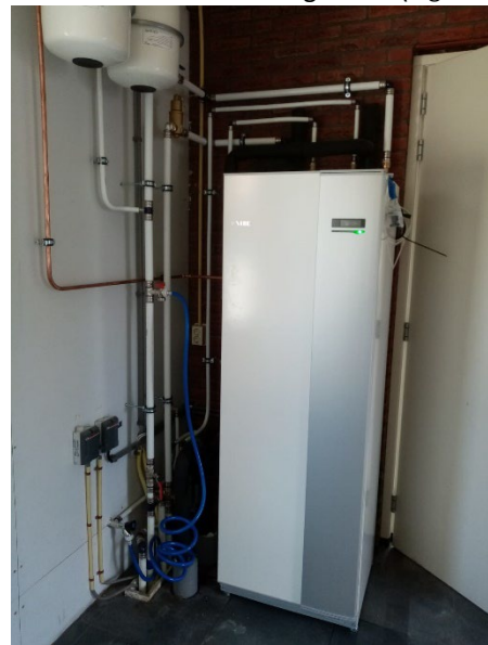
Figure 22. Ground source heat pump with integrated 180L DHW boiler (nefit-bosch, n.d.)
