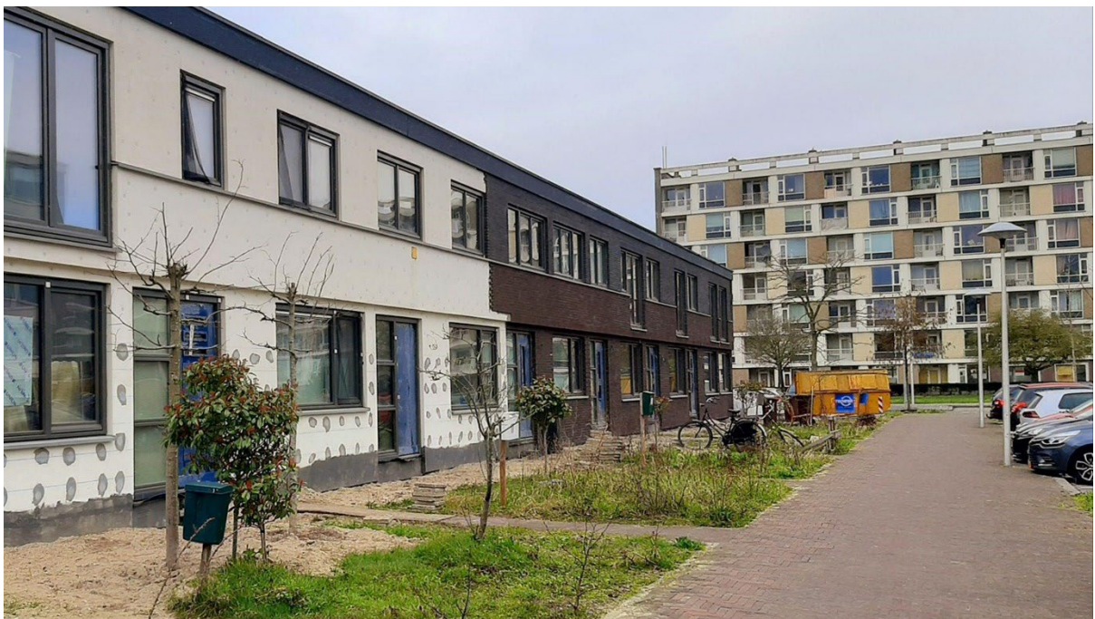
Figure 88. 10 private homes almost finished renovating
