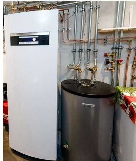
Figure 21. Ground source heat pump with integrated 180L DHW boiler + extra central heating buffer (nefit-bosch, n.d.)
