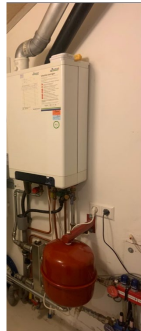
Figure 24. Hybrid heat pump (monoblock only) with only a hydraulic separator indoors (pdebonthbv, n.d.)
