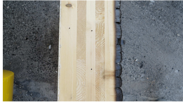
Figure 6.112 The char front progressed approximately 20 mm into the first layer of 40 mm thick CLT.
