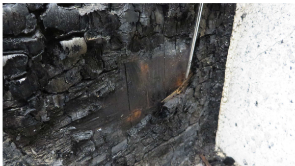
Figure 6.96 In the middle of the left side wall, the 1 st layer has fallen off. Removal of the charred 2 nd layer revealed the char front stopped at the interface between 2 nd and the 3 rd layer. Discoloured but otherwise unaffected wood of the 3 rd layer is visible
