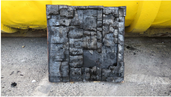
Figure 6.81 Various depths to which the charring front progressed and at which delamination and fall-off occurred.
