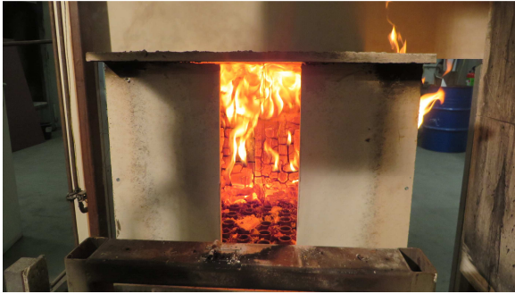
Figure 6.59 Removal of the heat flux sensor revealed the compartment in flaming combustion.
