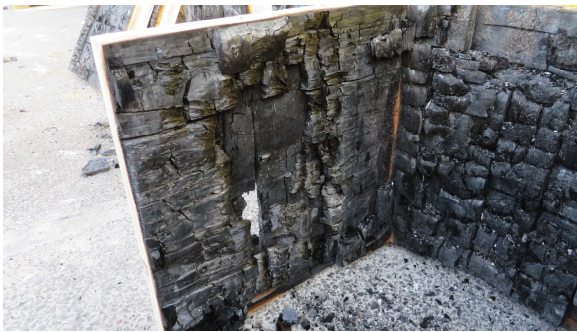
Figure 6.61 Various depths to which the charring front progressed and at which delamination and fall-off occurred.
