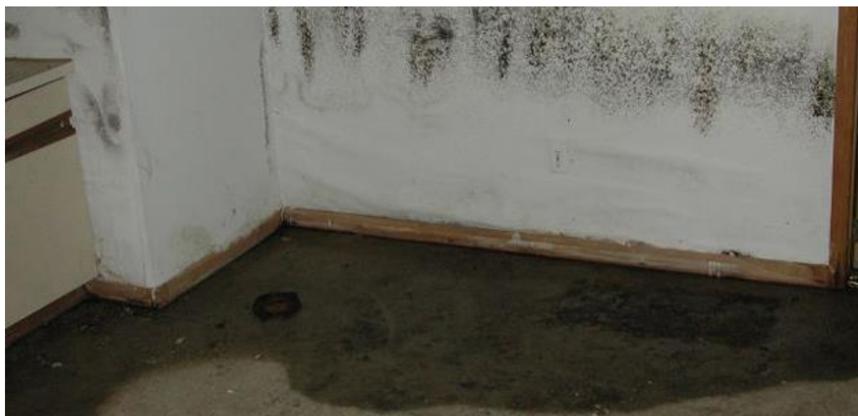
Figure 15: Small dewatering depth leading to rising damp that causes wet floors and walls (vochtproblemen-vochtbestrijding.nl)
