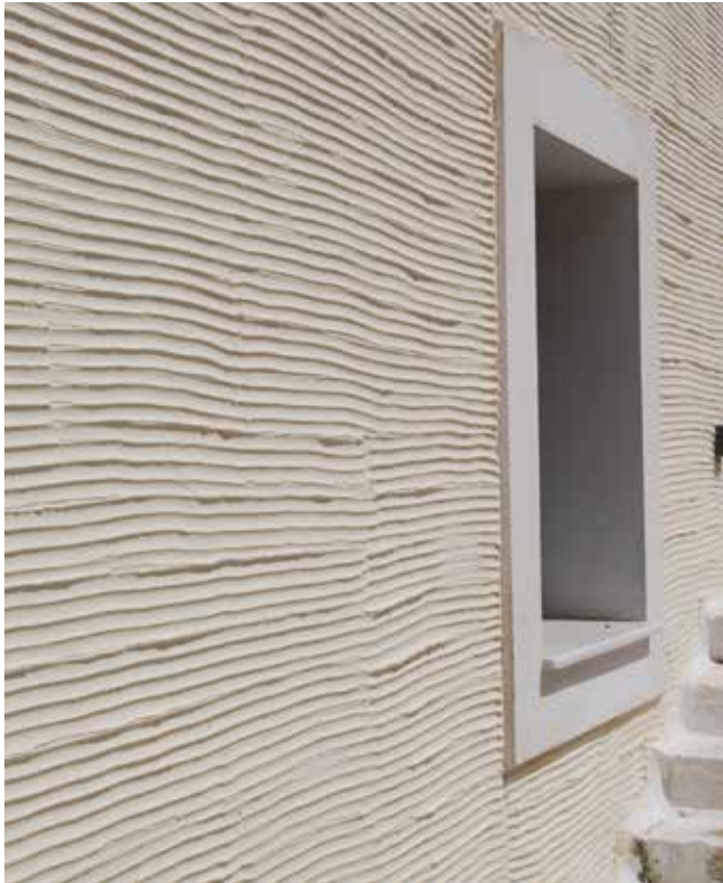
FIG. 3.13 Brushed plasterwork on a contemporary house on the Cycladic island of Andros, typical of the local tradition / Marieke Kuipers
