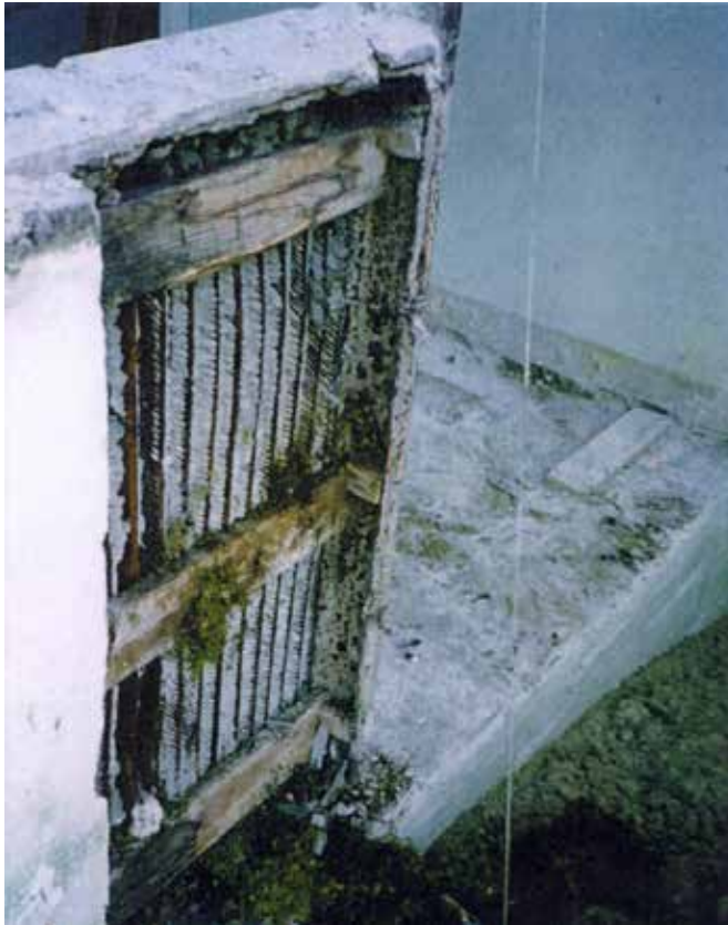
FIG. 5.9 'Destructive research' of an original part of the spandrel revealed wooden battens horizontally applied to the metal lattice (labelled as 'lath' in FIG. 5.7), which were not documented in any of the original drawings / Wessel de Jonge Architects
