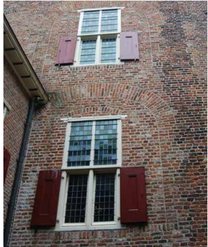
FIG. 3.14 Signs of weathering at Doorwerth Castle, the subject of a national debate in the Netherlands about its restoration that spanned the 20 th century / Marieke Kuipers
