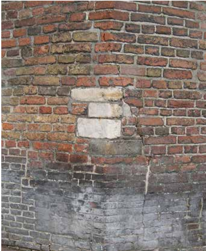
FIG. 3.15 Visible layers of repair in the wall of the medieval St Anthonis Gate, later reused as weigh house and place to demonstrate skills of brick laying for the guilds, Amsterdam / Marieke Kuipers
