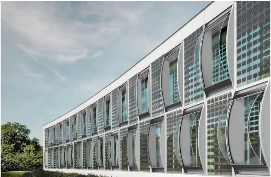
Figure 6: Rendering of case-study design of the proposed adaptive thin glass façade [Topcu, 2017]
