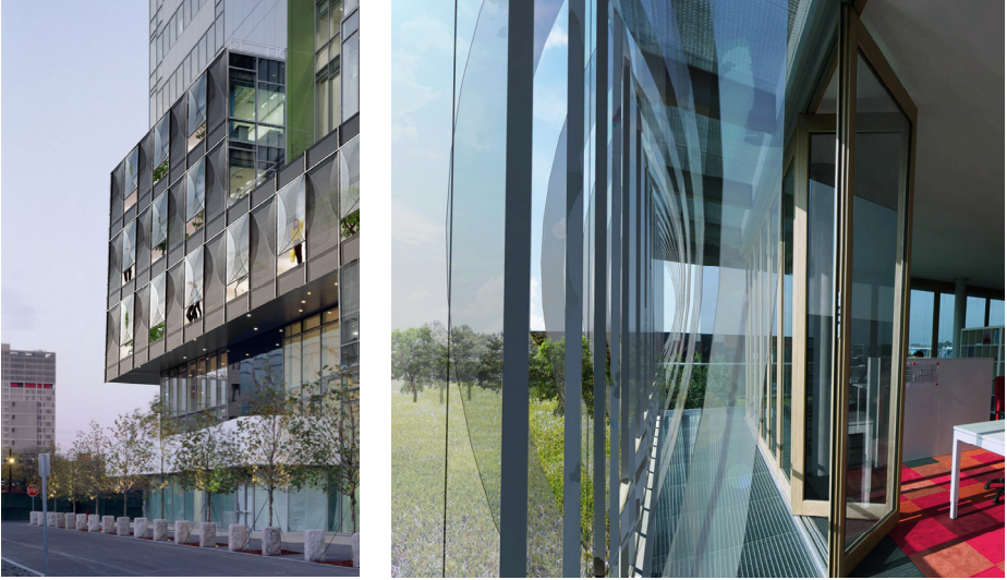
Figure 10: Case-study re-design of adaptive thin glass façade for the Genzyme Center [Miri, 2018]
