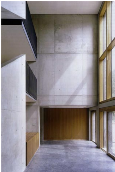
reference: C. Hendrich, A. Bauhofer, institute building in Freiburg, Germany (2005).
