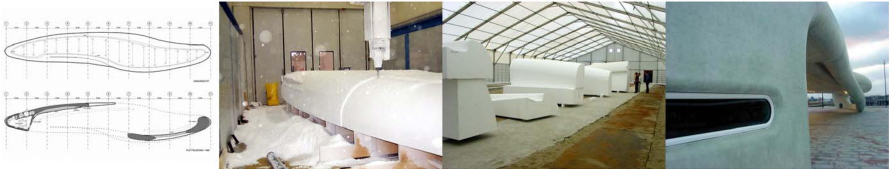
Fig. 2.12. Design, fabrication, assembly and final structure of 'The Amazing Whale Jaw' [<http://architettura.supereva.com>, April 2010]
