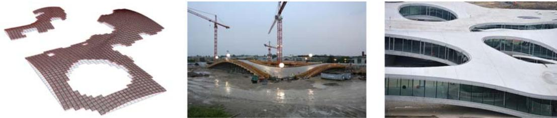
Fig. 2.13. A digital visualisation of the plans for all of the 1,500 formwork tables consisting of almost 10,000 CNC-cut individual cleats [<http://www.designtoproduction.ch>, May 2010], the construction site [<http://genevalunch.com>, May 2010] and the finished concrete shells [<http://davidgarciastudiomap.blogspot.com>, May 2010]
