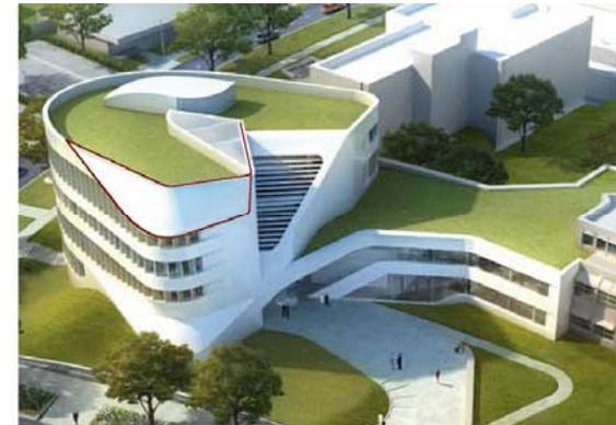
Fig. 7.4. Modelling the roof edge of the ZVE, Stuttgart by UNStudio with a ruling developable surface. Copyright left image: UNStudio
