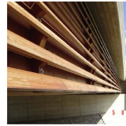
Figure 4.9: Adjustable slats can be applied on a truss (Simon and Koch, 2016)
