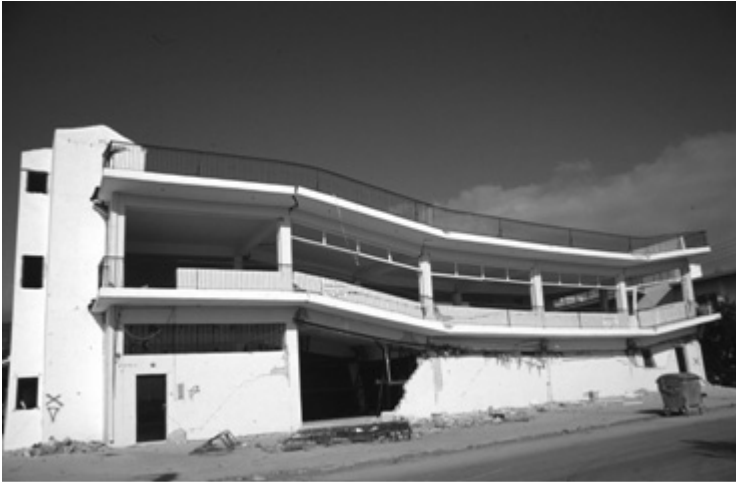
Damaged building by the Athens 1999 Earthquake, picture by P. Yannopoulos
