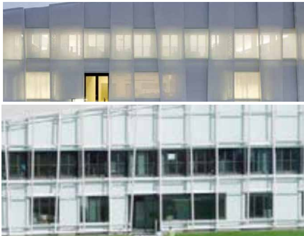
Title: Forschung Sedus Stoll AG Location: Dogern Designer: ludloff + ludloff Architekten Date: 2010 Medium: silicone-coated, glass fibre fabric
