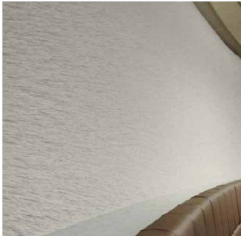
Title: Mercedes Benz museum Location: Stuttgart Designer: UNstudio & Inside Outside Date: 2006 Medium: concave brush wall. The brushesscatters the sound-waves gives better acoustics
